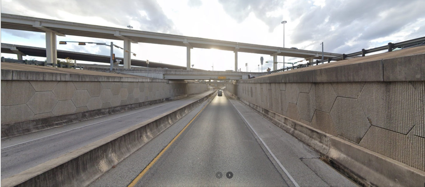
Figure 21. Lamar Boulevard Underpass north of Ben White Boulevard where the 1995/1996 cave survey projects the main cave passage of Airmen’s Cave leading to the Formation Room passes beneath. According to the 1974 cave map, the same passage passes under the underpass on the opposite side of this intersection. The posted depth of the underpass is 16 feet 6 inches (photo credit: Google Maps 2021).
