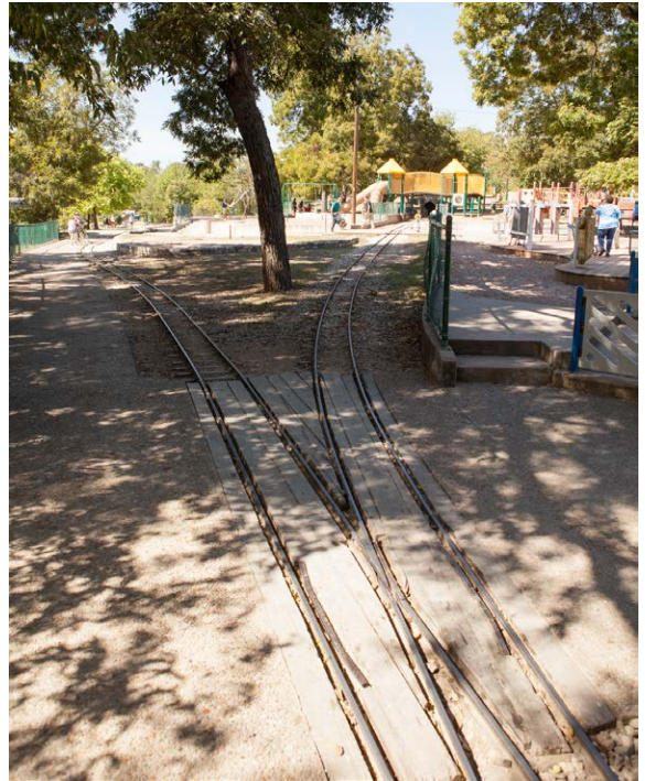
Zilker Train: The Zilker train has been in service since the early 1960s. The track, which is visibly irregular and variable in gauge, appears to be approaching the end of its serviceable lifespan.
