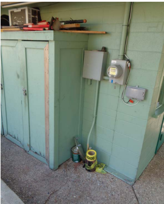
Zilker Train: Deficient storage, as here at the train depot, is a common throughout the Bathhouse Zone.
