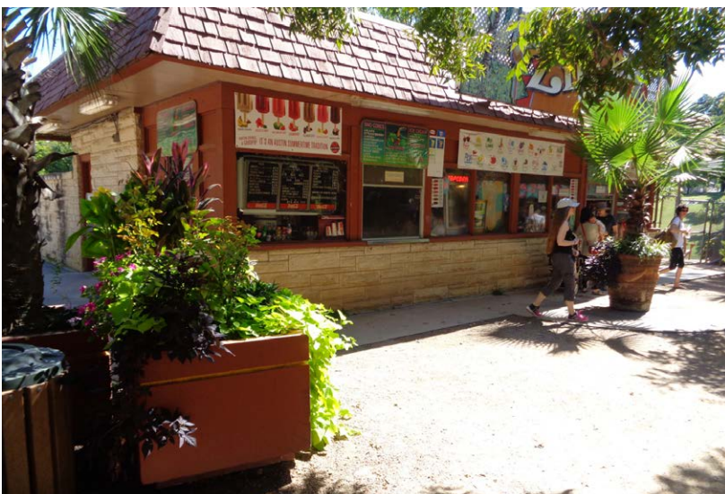
Zilker Café: The fabric of the Zilker Café dates to the early 1960s, when it was constructed to replace a predecessor damaged beyond repair by flooding.
