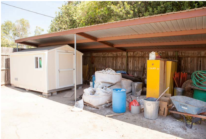
Maintenance Yard: Ad-hoc storage is characteristic of the current Maintenance Yard. The storage of fuels and other chemicals within the yard over the decades raises concerns over the viability of any potential re-purposing of this facility.
