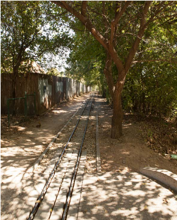
Zilker Train: The right-of-way allocated to the Zilker train leaves an excessively narrow pathway between the track and the enclosure of the maintenance yard.
