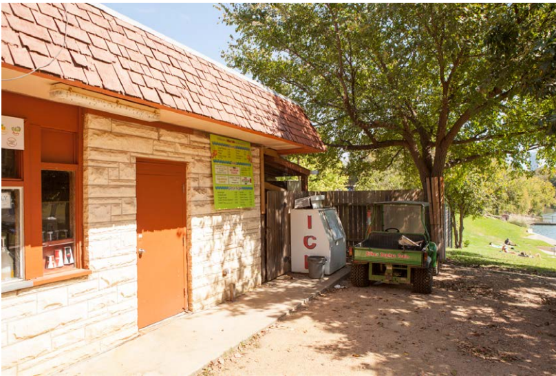
Zilker Café: Due to inadequate building area, the operators of the Café rely on exterior and off-site storage. The area shown here used for vehicular parking and storage is within the pool enclosure and drains into the pool.
