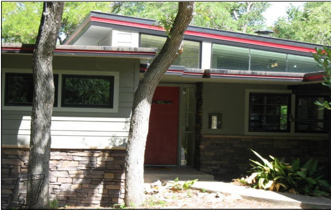
Several houses in the Zilker neighborhood are still recognizable as Stenger creations, like this one on Bluebonnet, with its low roof, clerestory windows, and stonework.
