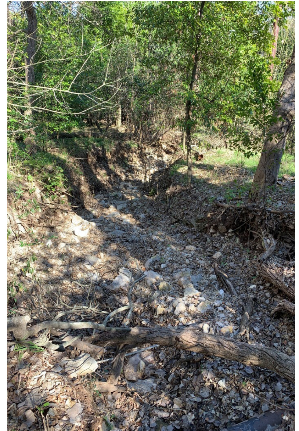
Gully erosion located between Stratford Drive and Lady Bird Lake.
