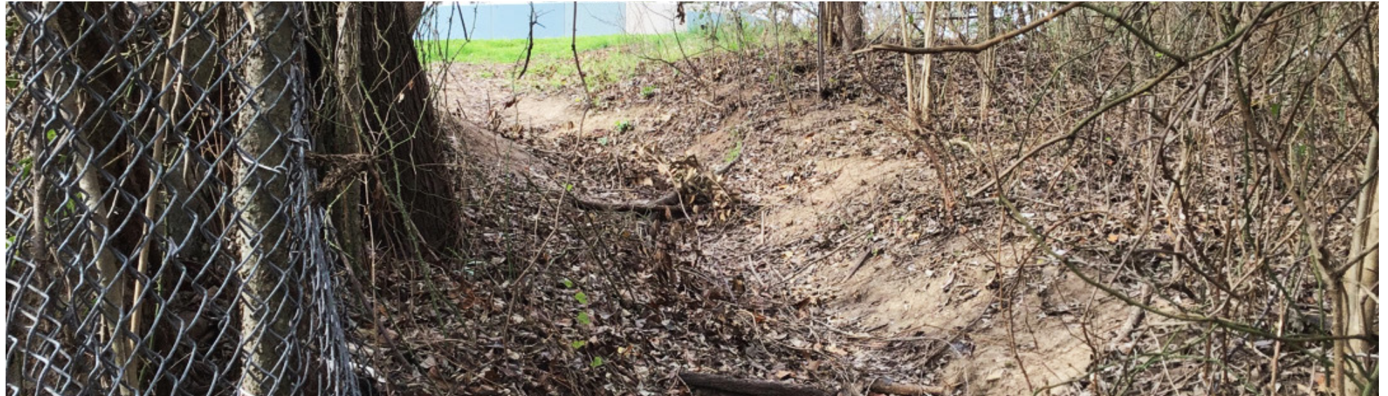
Gully erosion forming from stormwater off paved areas
